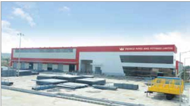
JOBNER - RAJASTHAN PIPES & WATER TANKS
