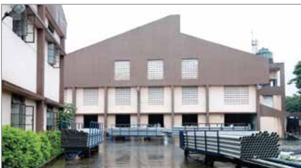
DADRA - SILVASSA PIPES & WATER TANKS
