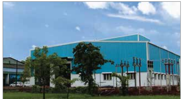
KOLHAPUR - MAHARASHTRA PIPES
