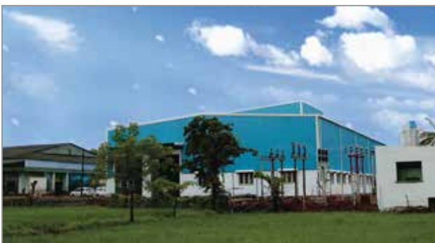
CHENNAI - TAMIL NADU PIPES
